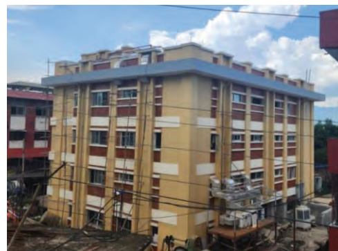
Figure 3: OT block in Bhaktapur Hospital
