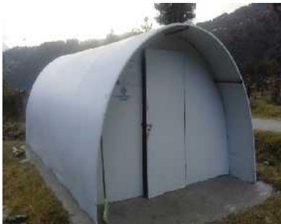
Transit Home, store room for PT equipment.
