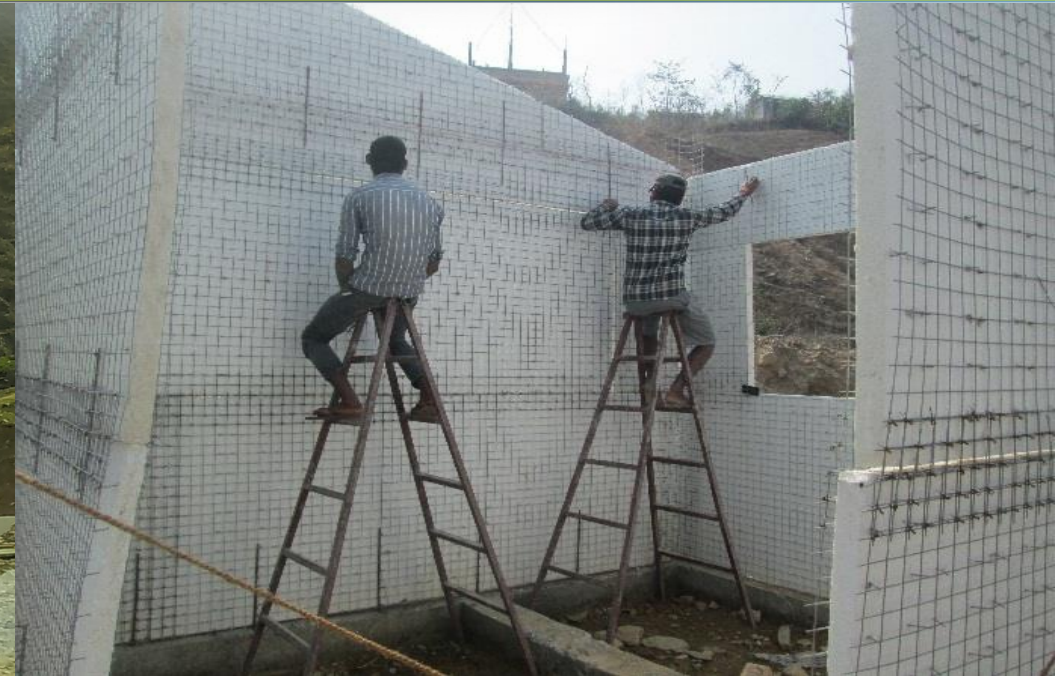
Manthali PHCC (OCMC, OT, Diagnostics) in 3D Panel Systems
