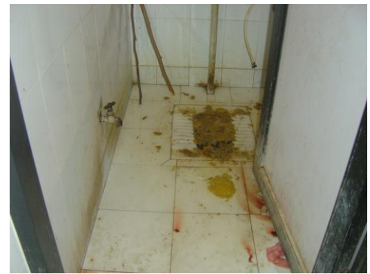
Photo: Poorly managed toilet at maternity ward of the hospital
