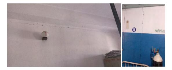
Figure 9: Cracks in walls
