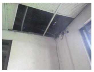
Figure 16: False ceiling of Emergency block
