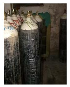
Figure 13: Oxygen Cylinder Kept Unbraced
