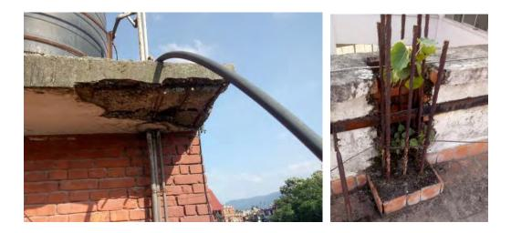
Figure 8: Corrosion in Main and Maternity blocks
