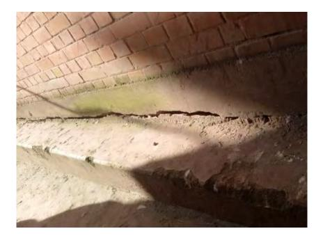
Figure 11: Settlement cracks in Maternity Block
