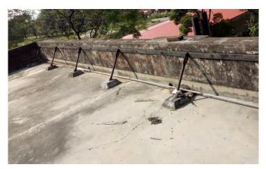
Figure 14: Parapet wall achorage
