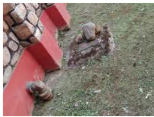
Figure 18: Foundation Exploration of Masonry Block
