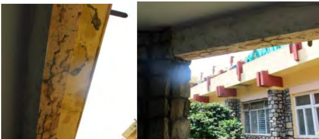
Figure 5: Corrosion cracks in Emergency Block & OPD Block
