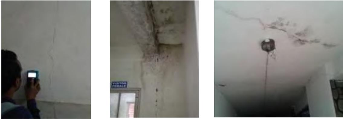
Figure 8: Vertical Cracks on Masonry Wall (Sealed area of Seismic Separation)
