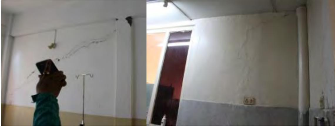
Figure 6: Wall cracks in Emergency Block & OPD Block
