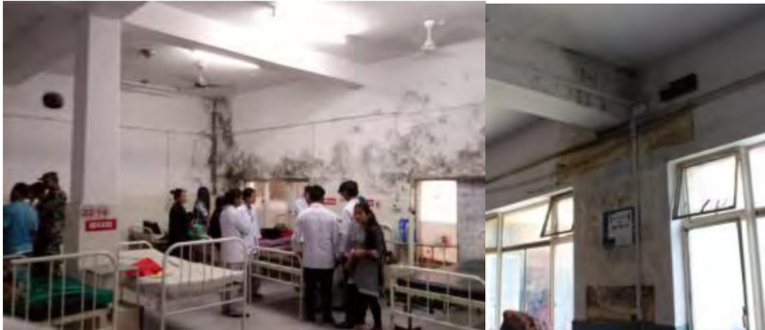
Figure 4: Serious seepage issues inside Emergency Block & OPD Block
