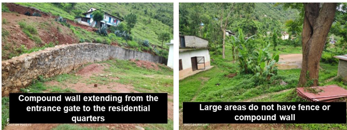
Figure 13: Inadequate boundary wall and fence
