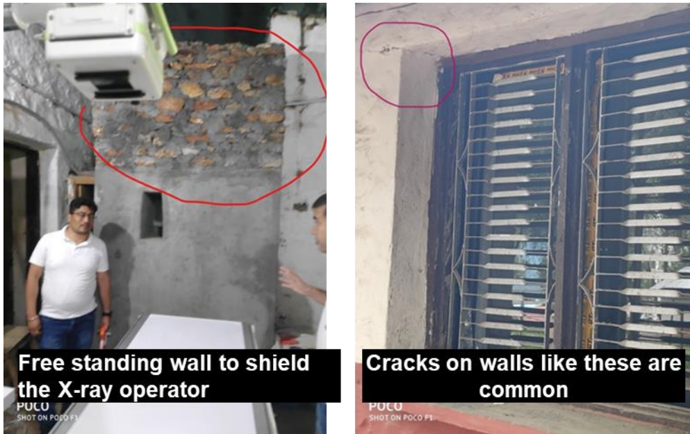
Figure 15: Defective brickwork
