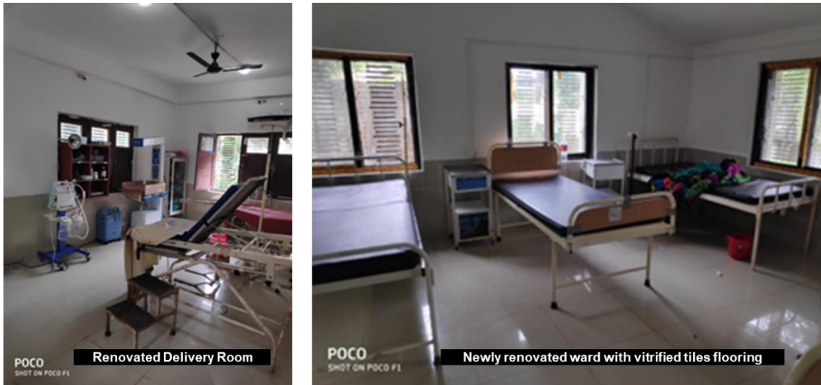
Figure 4: Renovations and floor improvements
