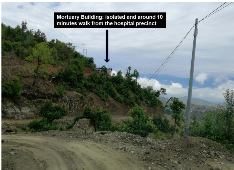
Figure 7: Dullu Hospital Mortuary Block
