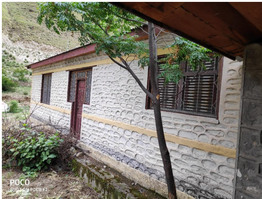
Figure 14. BEOC building without HVAC (Photo from rear of the hospital)
