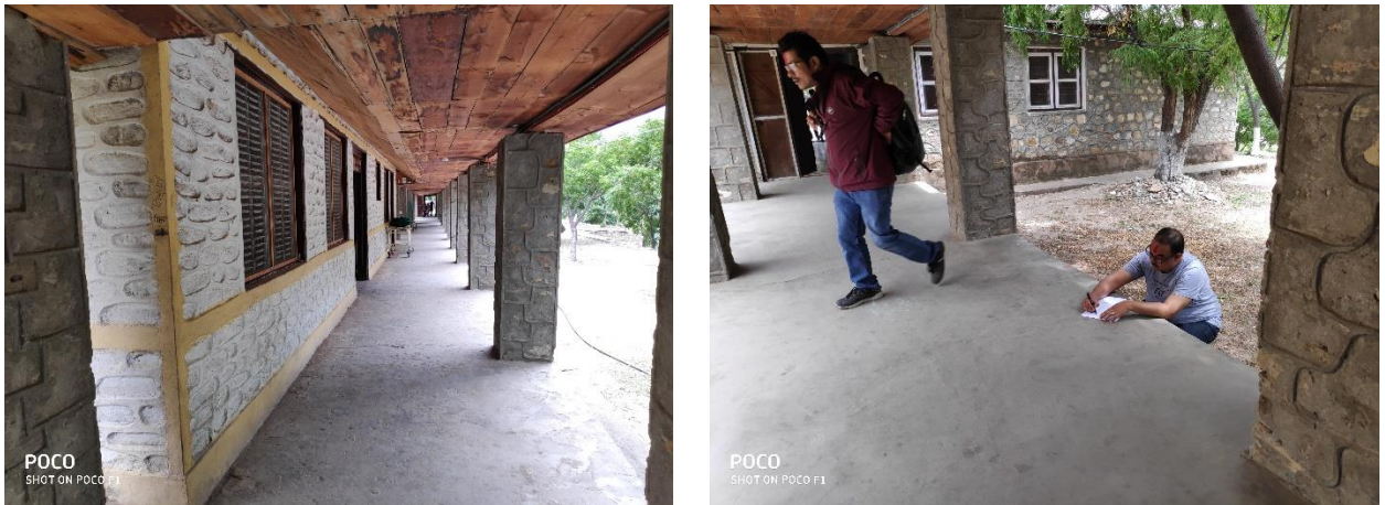
Figure 18: Exterior walkway floor surface
